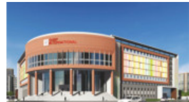
Snbp Chikhali New Building 2026
